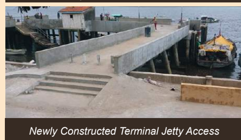
Newly Constructed Terminal Jetty Access and repaired Lamu Seawall
