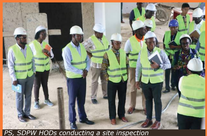
SPDW, LVBC and the contractor team during a joint site inspection activity
