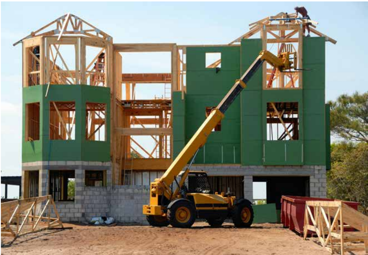
Figure 5-12: Timber and Masonry Construction
