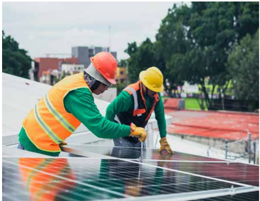
Figure 5-8: Solar Panel Installation
